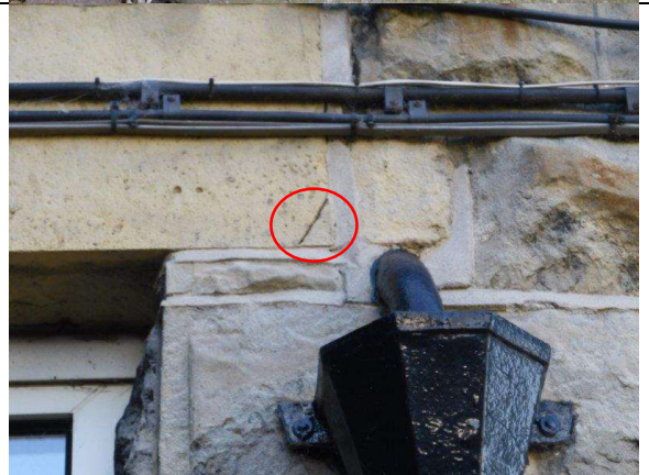
A hairline crack to the bottom right-hand corner of the lintel on the kitchen window outside the back door.
