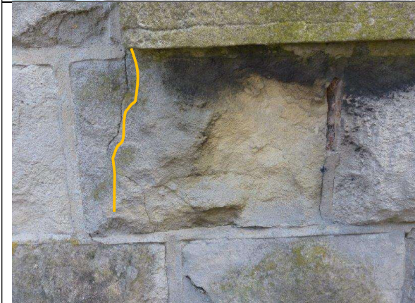
A hairline crack to the bottom right-hand corner of the lintel on the kitchen window outside the back door.
