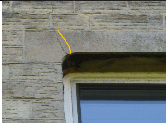
Bedroom two down to the drawing room – gable end – hairline stepped cracking on the wall and through the lintels. This should be recorded, repaired and monitored.
