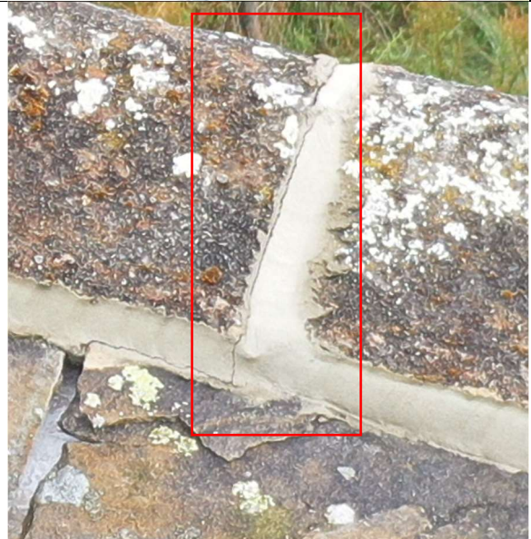
Ridge – example of a hairline crack to the pointing detail.
