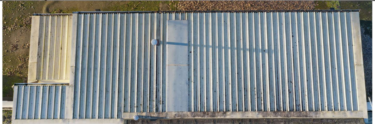
Overhead photo of the roof.
