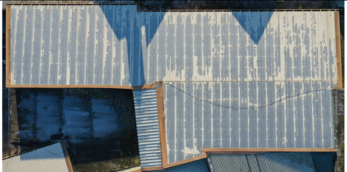
Overhead photo of the roof pitches.
