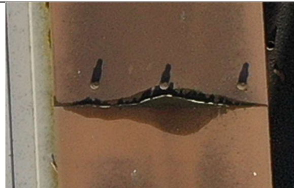
Example of some light corrosion on the cappings. This should be treated in the short term to prevent further deterioration.
