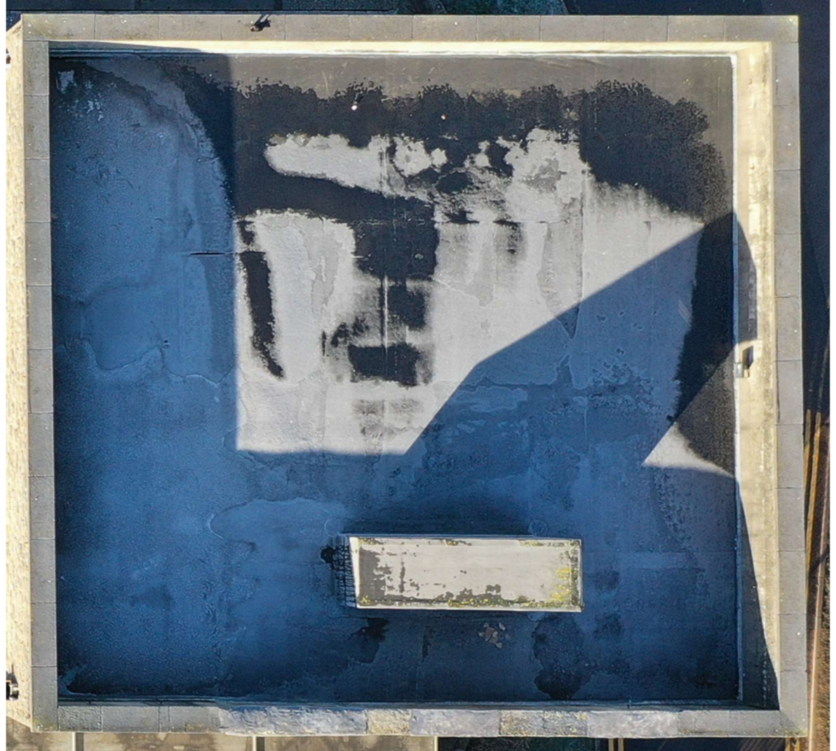
Overhead photo of the tower roof.
