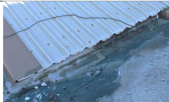
Example of some light corrosion on the cappings. This should be treated in the short term to prevent further deterioration.
