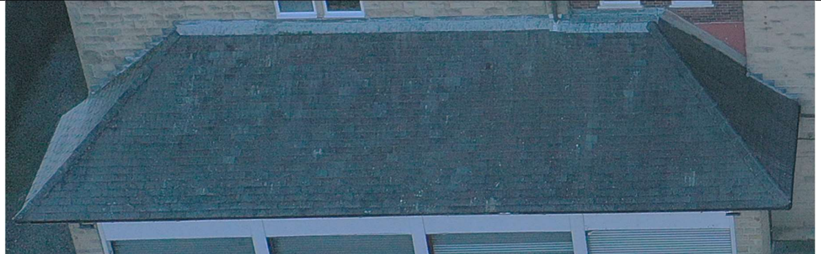
Overhead photo of the roof.
