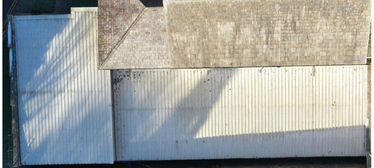
Overhead photo of the roof.
