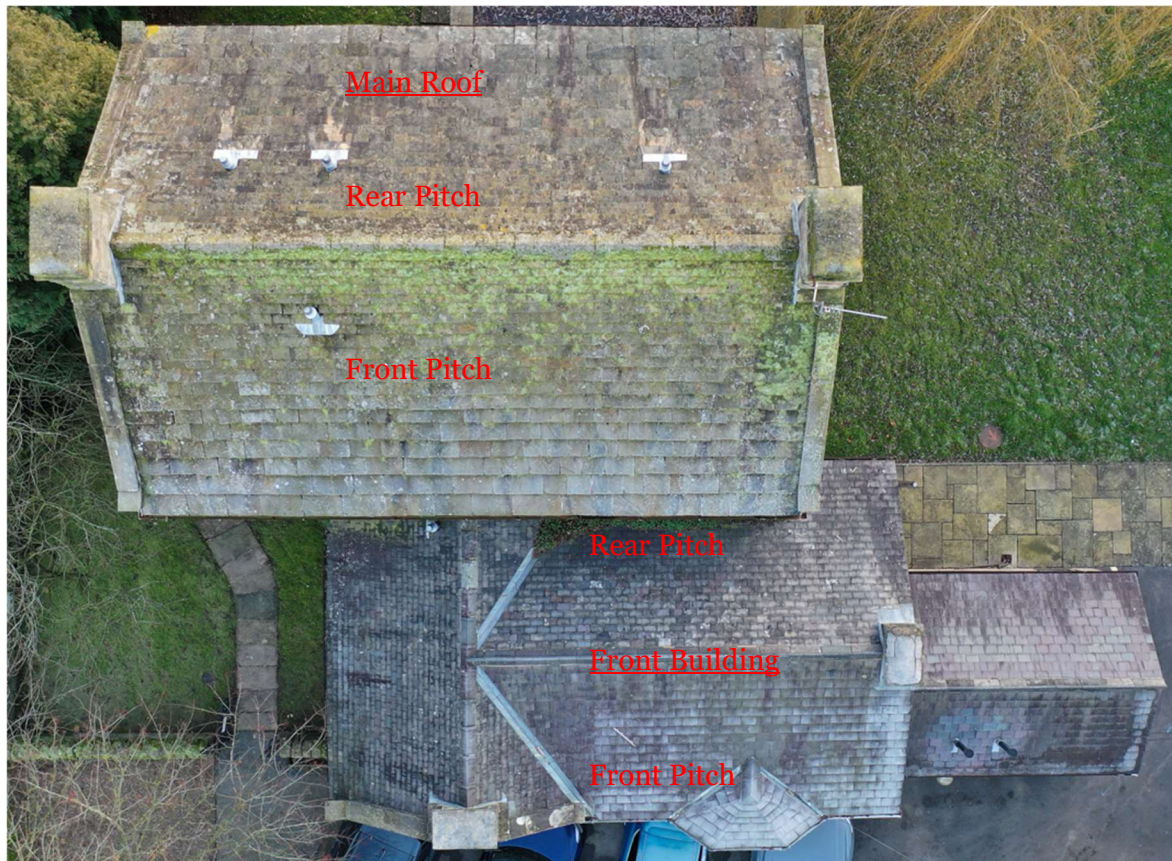
Overhead photo of Roof N.
