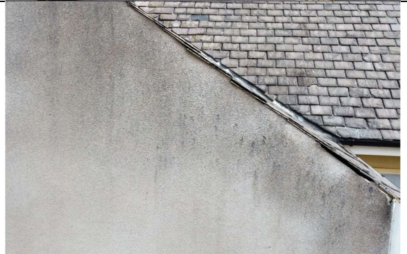
Off-shot, rear elevation – the verge line is stained due to the abovementioned lack of projection on the verge slates.
