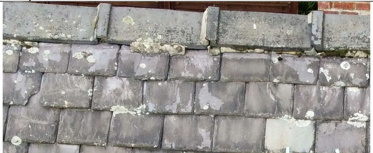
The areas of slipped, missing and damaged slates need to be repaired immediately. Example photos are below.
