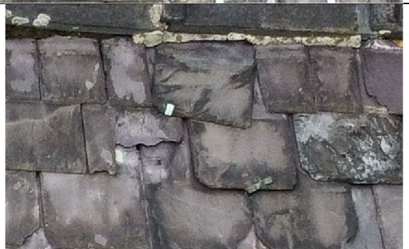
The areas of slipped, missing and damaged slates need to be repaired immediately. Example photos are below.
