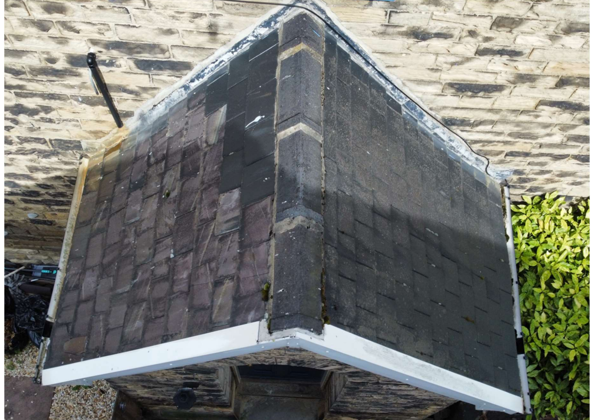
Overhead photo of the porch roof
