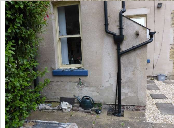
Off-shot, rear elevation – the verge line is stained due to the abovementioned lack of projection on the verge slates.
