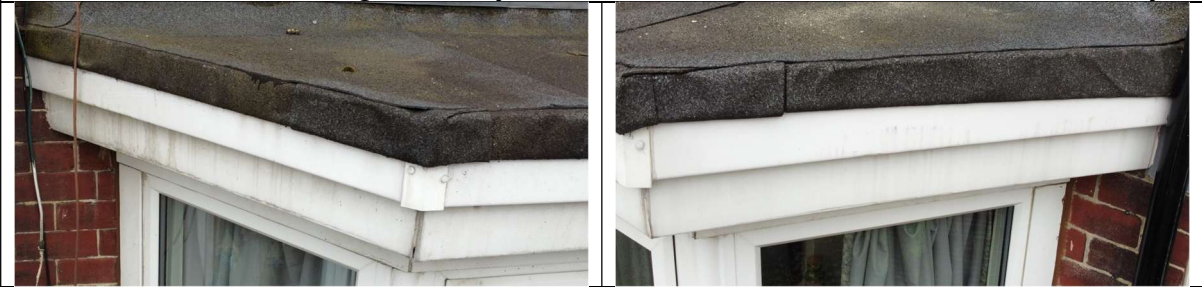
The felt is ruckled and not particularly well detailed around the front and sides of the bay.
