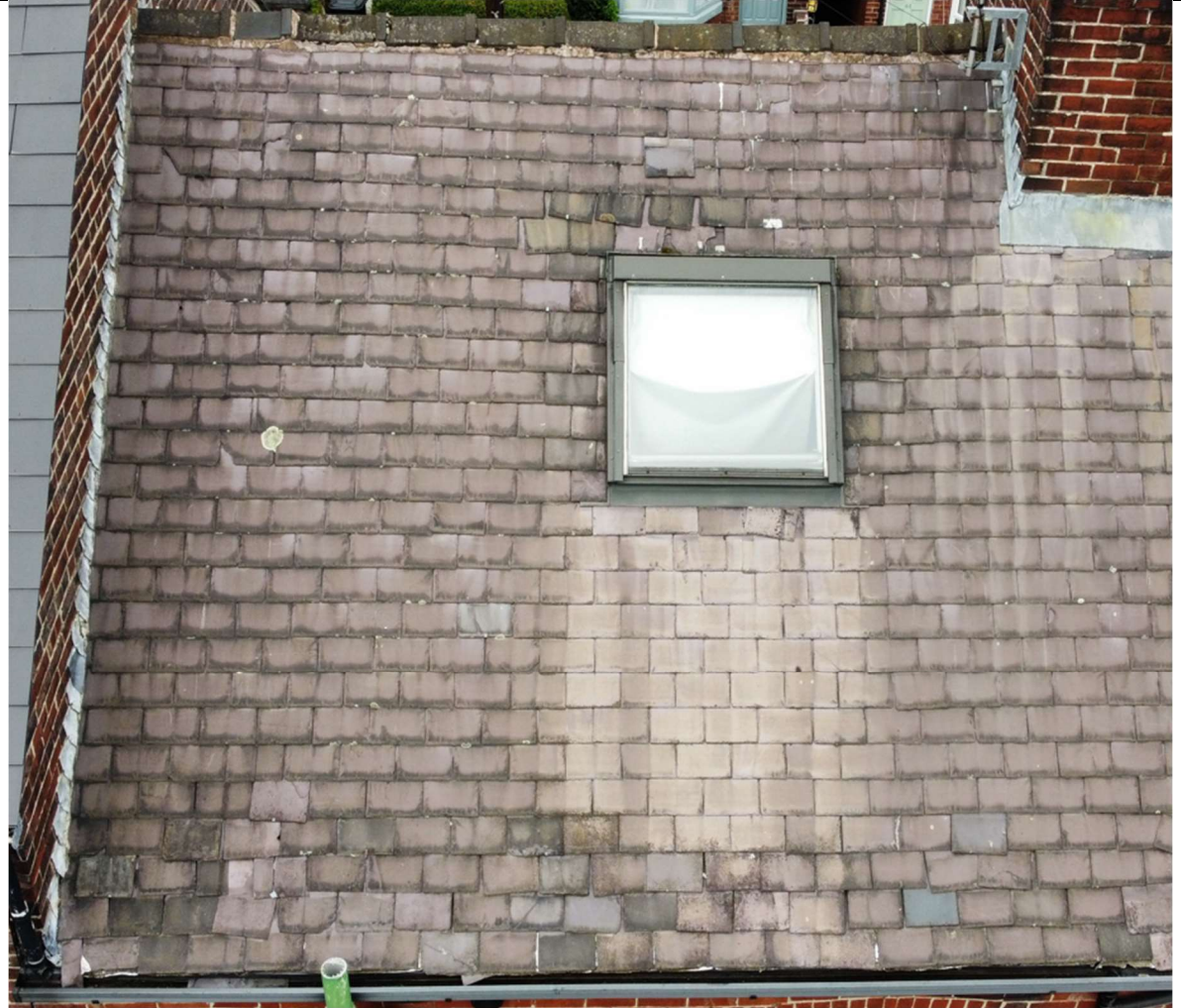
There are several areas of damaged slates across the pitch. All areas of damaged slates should be repaired/replaced as soon as possible. We have included some example photos of the areas below.
