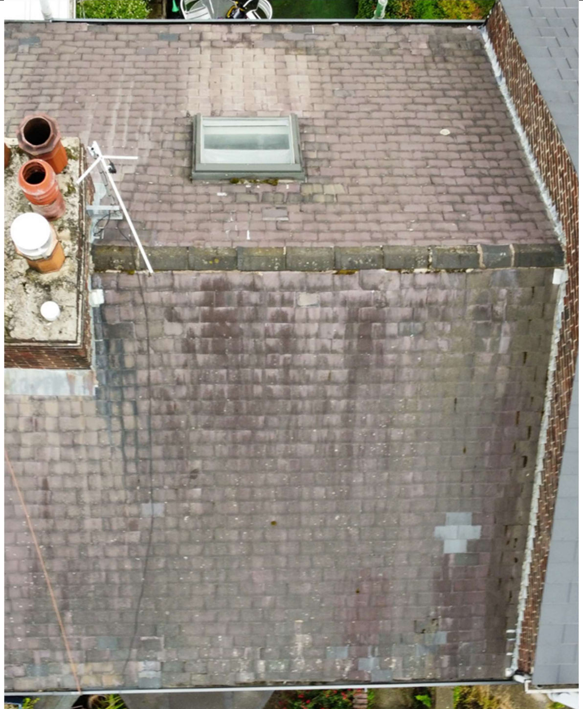
Overhead photo of the front and rear roof pitches.
