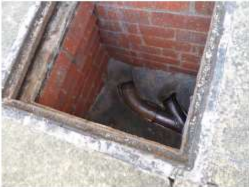
Manhole to side of property
