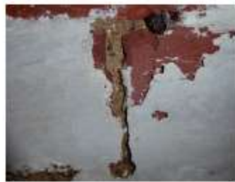
Softer mortar than cement – white flecks visible likely to be un-slaked lime
