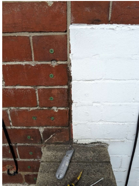
Fig. 15 – Pointing to the party wall above the front LHS boundary wall.
