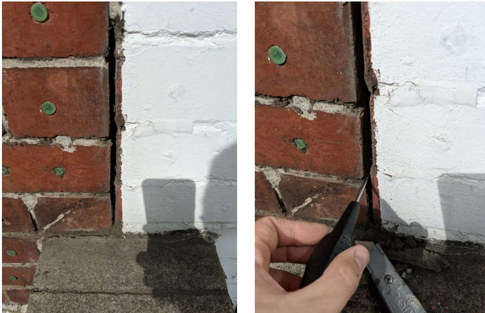
Fig. 22 – Silicone removal to reveal exposed joint.
