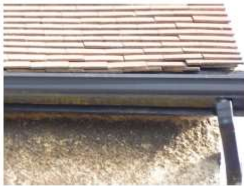
Square downpipe connecting into round gutter
