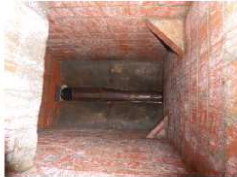
Manhole to front of property
