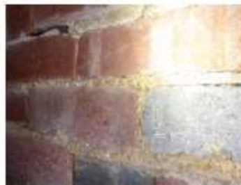
Softer mortar than cement – white flecks visible likely to be un-slaked lime
