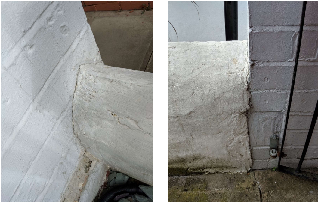
Fig. 18 – The RHS front boundary wall abuts the front elevation.
